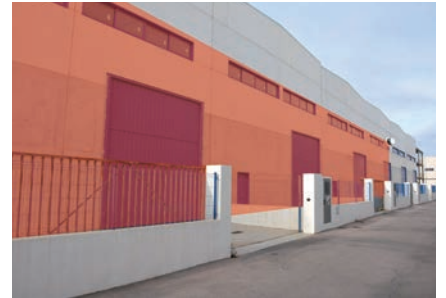
Wall protection (outdoor) at Warehouse
